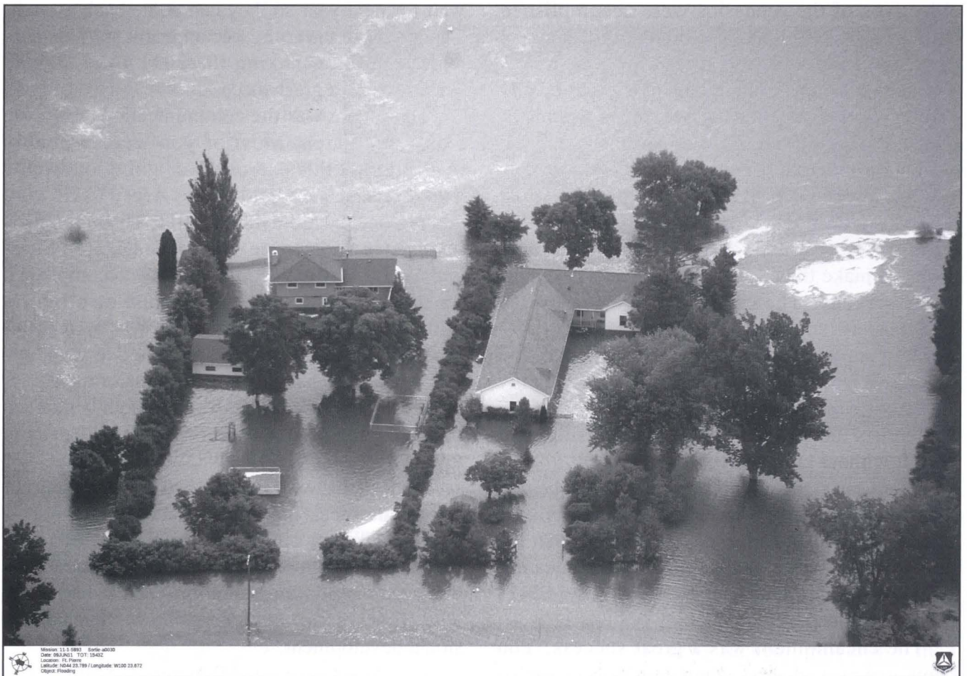
For some South Dakota homeowners and businesses along the Missouri River, despite the best efforts of the Civil Air Patrol, the National Guard, the State of South Dakota, FEMA, and other state and local agencies, the flood fight was lost. Here, homes north of Ft. Pierre, S.D. succumbed to the force of the Missouri River. Photo by Capt. Jerry Foy.
